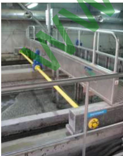
➔ Degritting and degreasing suction bridge for rectangular basin
