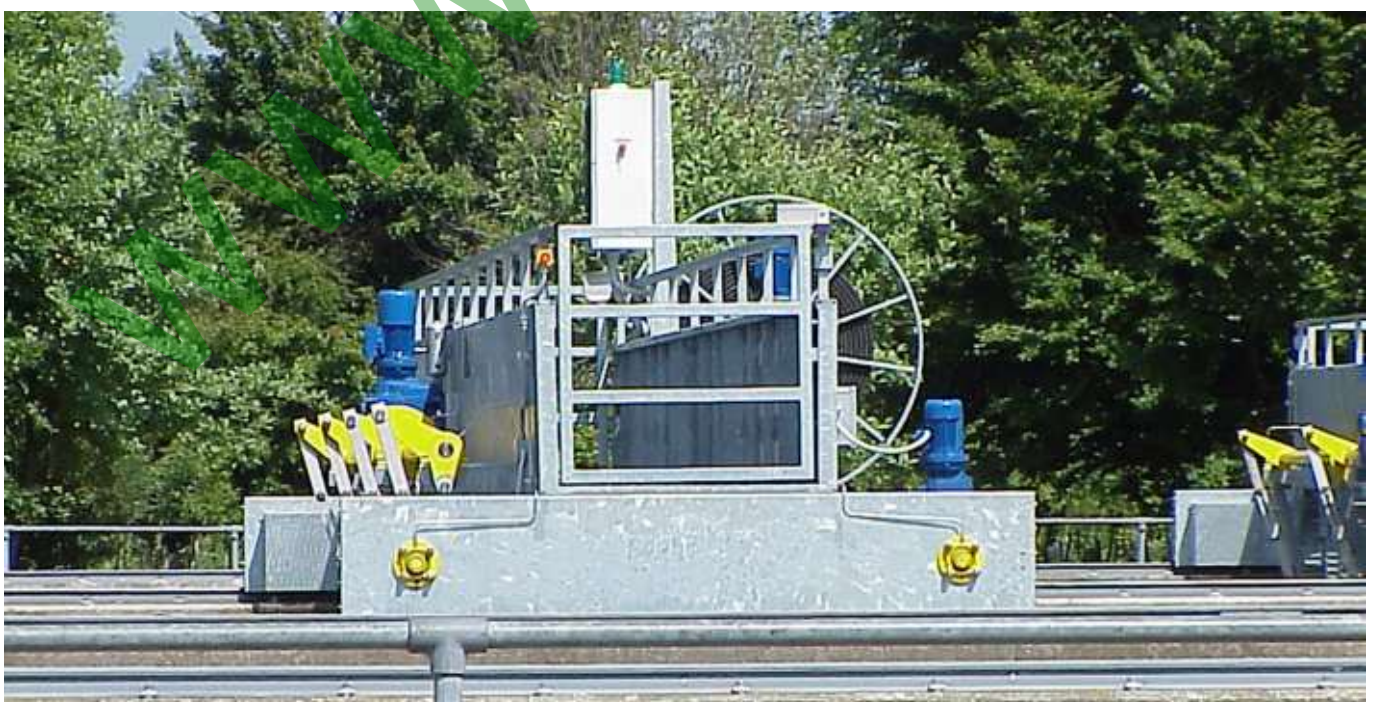
→ Backward and forward scraper for rectangular decanter
