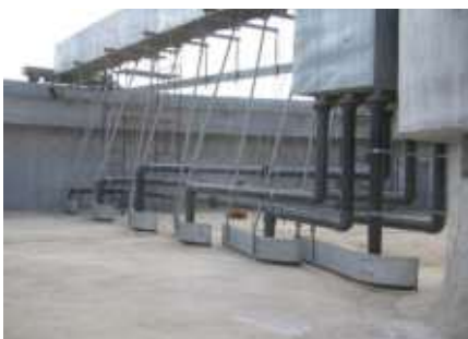
→ Peripheral drive aspirated scraper for circular decanter
