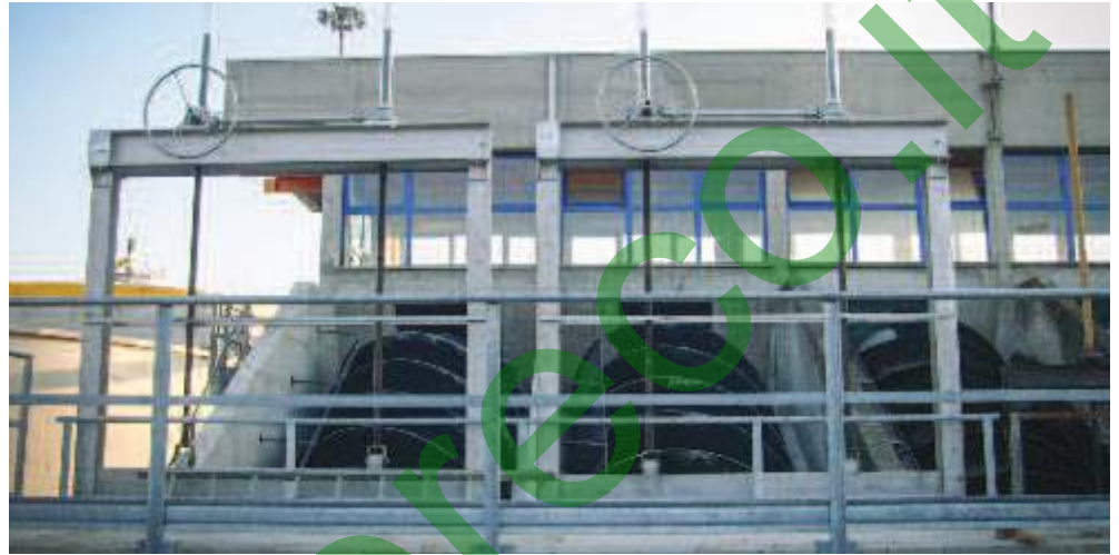
SERECO penstocks, P2V3 model, installed at IDAR BOLOGNA Municipal WWTP in Italy
