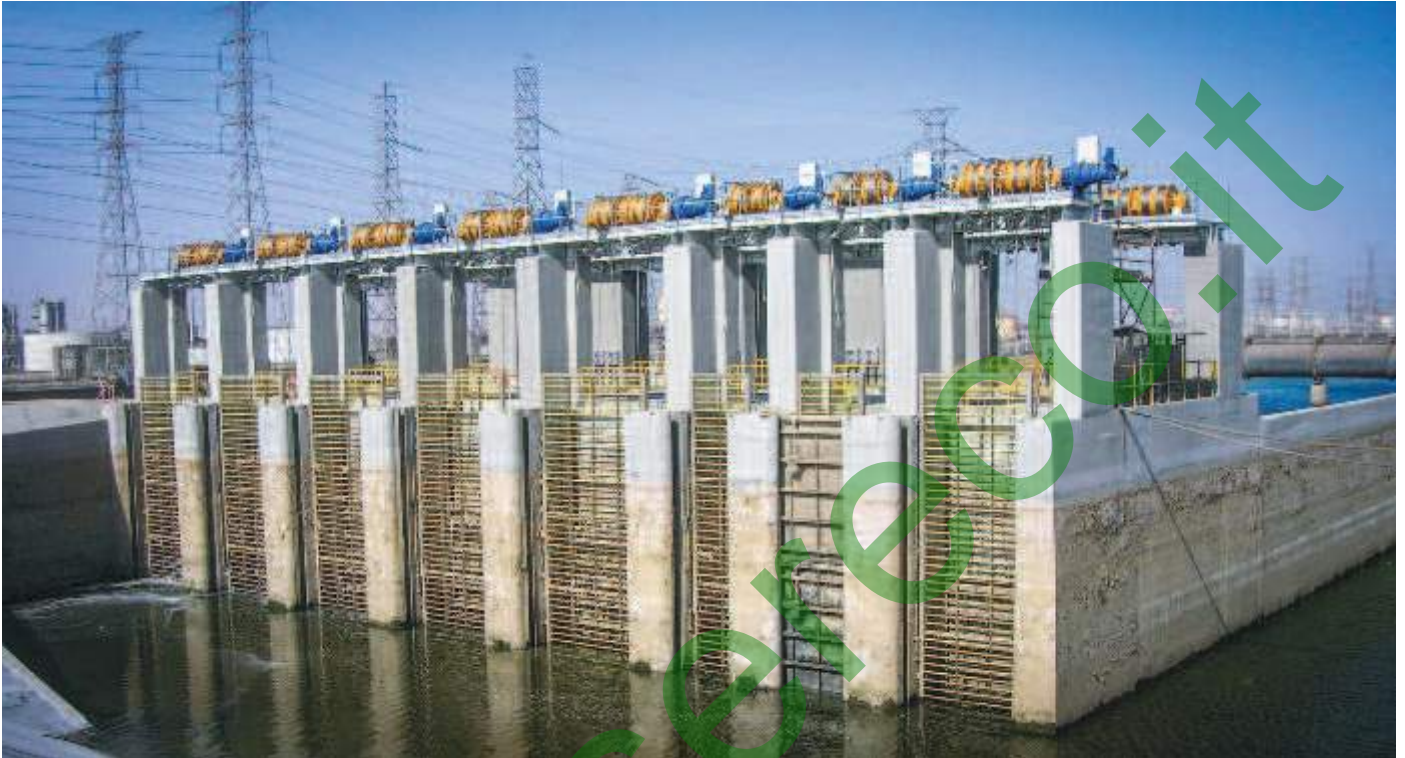
SERECO penstocks, P2V4 model, various series, installed at Jubail seawater intake in Saudi Arabia
