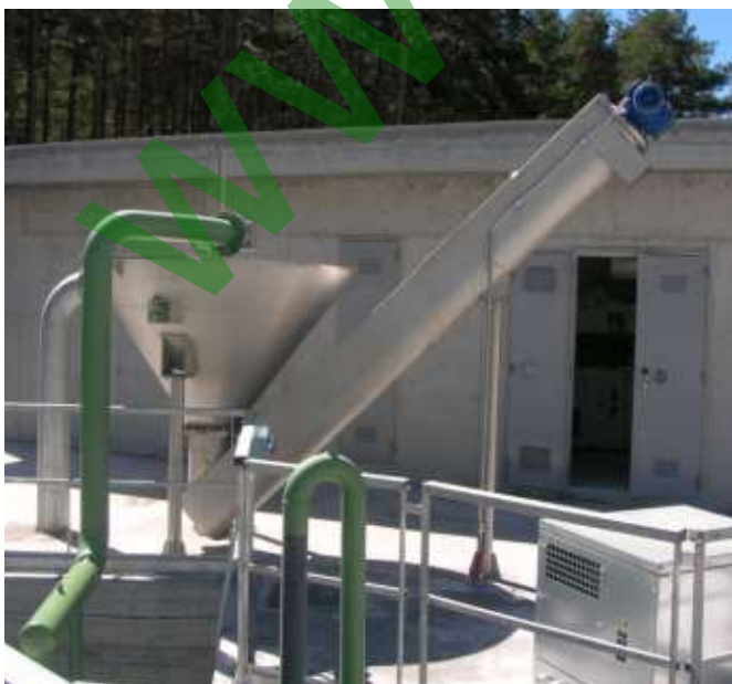
→ Screw grit classifier with integrating Coanda effect
