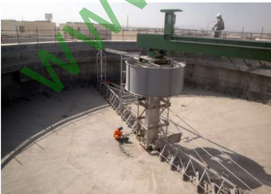
➔ Scraper for circular decanter with central control
