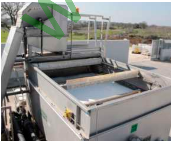
→ GRS drum screen installed
