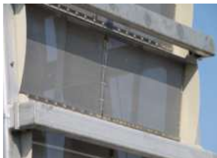
→ Detail of a belt screen dual flow GNAFO1
