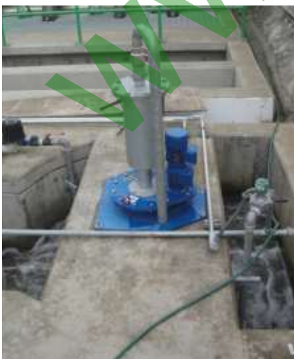
→ Rotating blade grit remover
