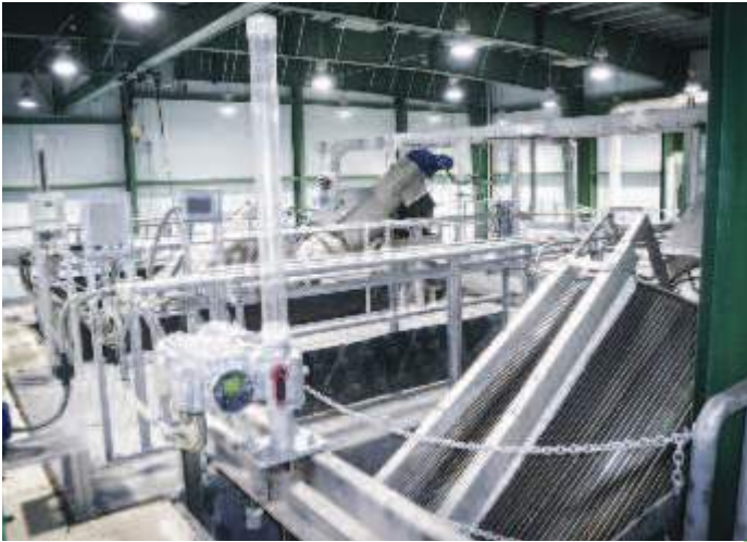
SERECO penstocks, PV4 model, installed at KAUST WWTP in Saudi Arabia
