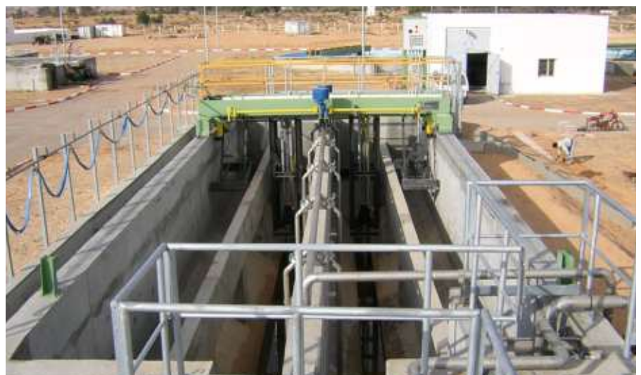
➔ Degritting and degreasing suction bridge for rectangular basin
