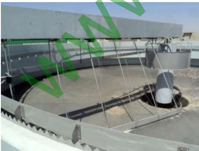
➔ Peripheral drive scraper for circular decanter
