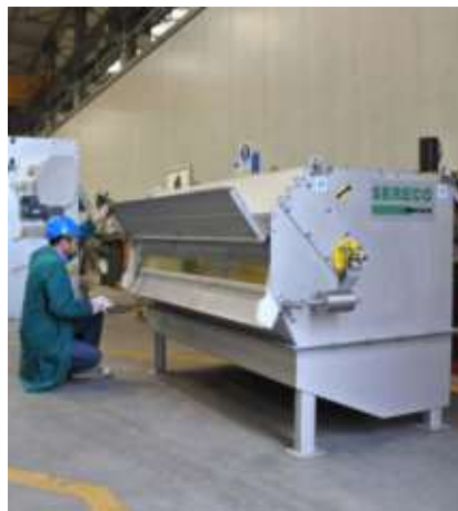
→ GRS drum screen installed
