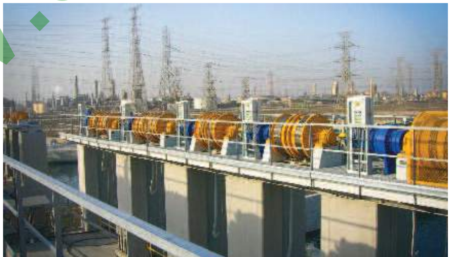
SERECO penstocks, P2V4 model, various series, installed at Jubail seawater intake in Saudi Arabia
