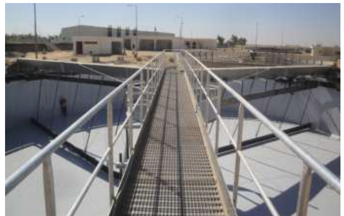
➔ Scraper with peripheral drive with three arms for circular decanter
