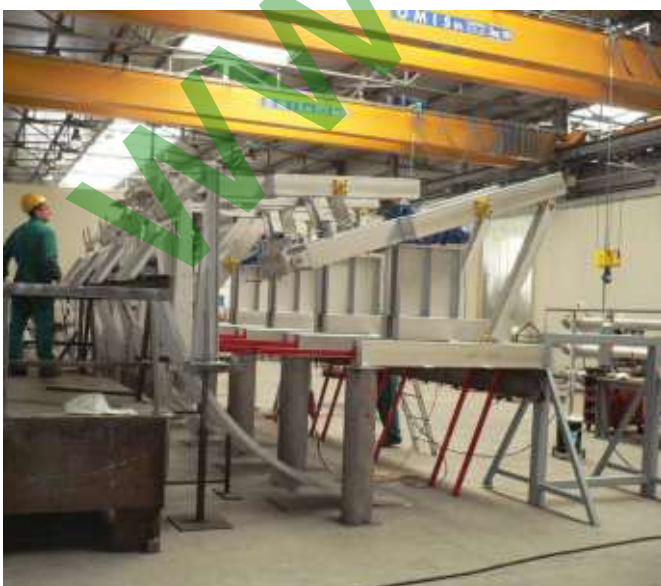
➔ Group of 4 GCMR being tested
