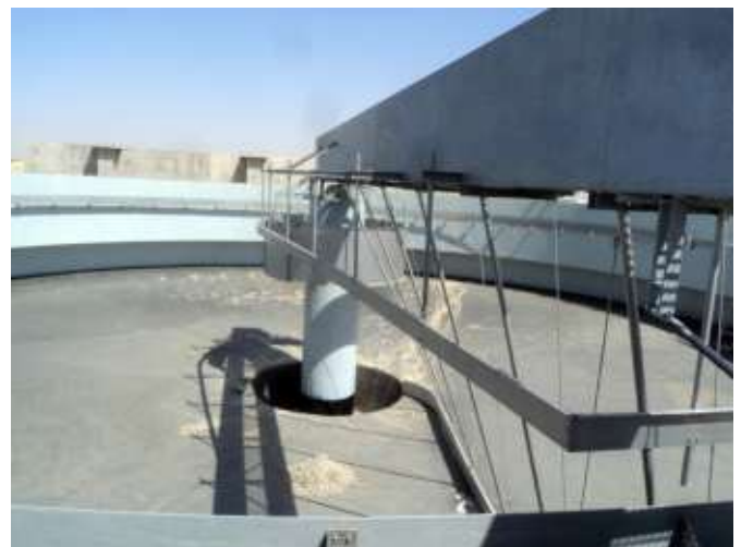
➔ Peripheral drive scraper for circular decanter
